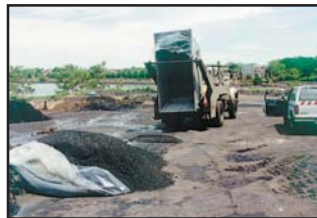
Lugger and Dewatered Grit
