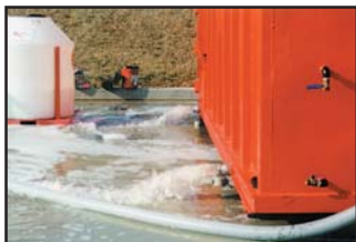
Clear Water from Sludge Mate®
